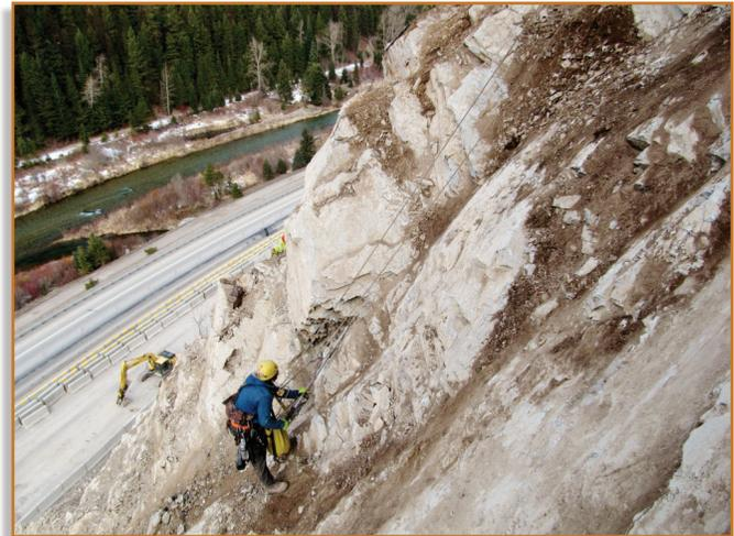
Rope access for I-90 MP 22 rock slope emergency response
