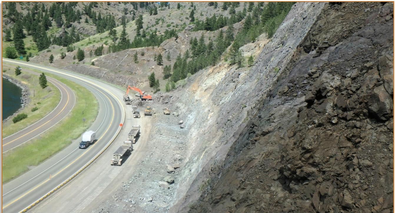
Controlled highway blasting techniques on the I-15 (D3) rock slope corridor
