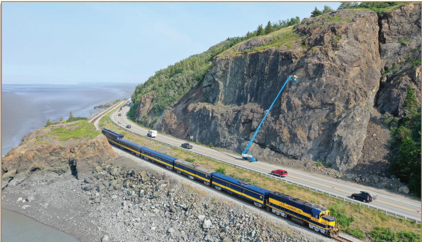
Boom-lift rock slope assessment and traffic control along Seward Highway in Anchorage
