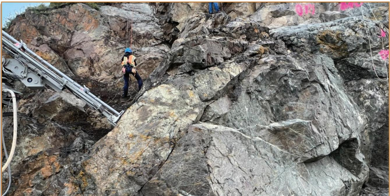
Construction layout via rope access and drilling for rock bolt installation on the Seward Highway rock slope corridor
