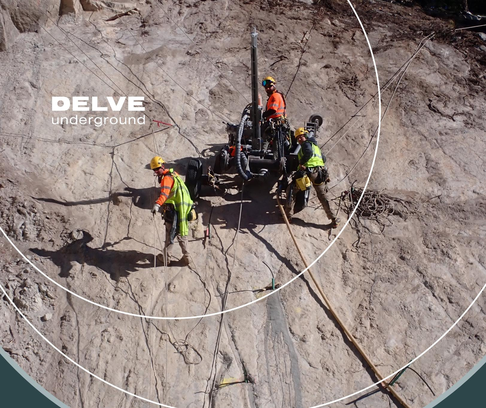
An aerial photograph of a construction site on a steep, light-colored rock face. Three workers wearing high-visibility vests and hard hats are positioned around a large, vertical drilling rig. One worker is on the rig, another is to the left, and a third is to the right. Ropes and cables are visible across the rock surface. The scene is framed by a white circular arc.
