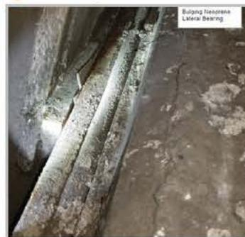
Pier 18’s bearing is compressed, which means that the bridge cannot move as it should. Instead, the bearing is creating additional pressure on the surrounding area and affecting the bridge as a whole.
