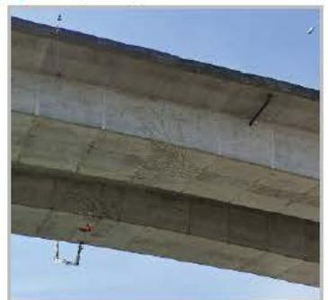
Potentially dangerous cracking was discovered in the center of the bridge, both inside and outside the structure, leading to its closure. The Pier 18 bearing likely contributed to the cracking.
