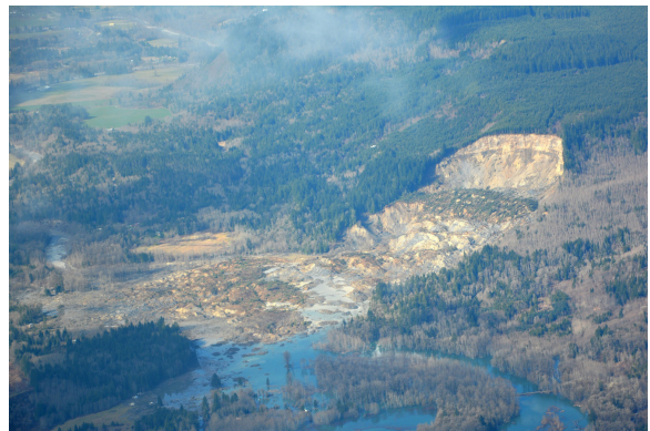
Top: construction underway on SR 530 following devastating Oso landslide (Bottom).
