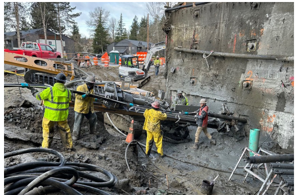
Construction of the tieback wall for fish passage below I-405.
