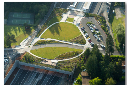
Evergreen Point Land Bridge over SR520 (DEA/HBB)
