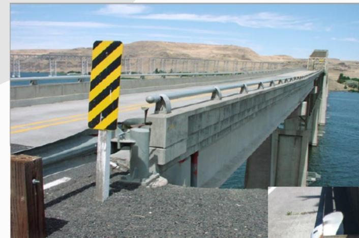
The Type 3 anchor was primarily used at bridge ends. This anchor consisted of a steel pipe mounted vertically in a concrete foundation. Bridge approach guardrail was then mounted on the steel pipe.
