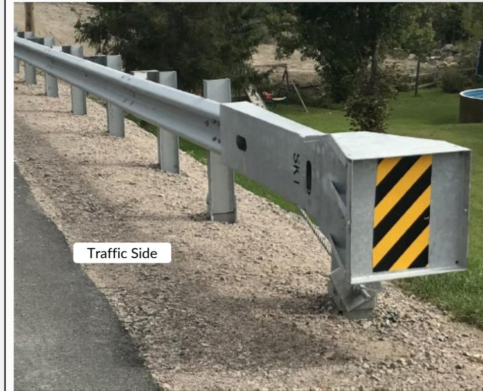
The manufacturer allows damaged NCHRP 350 SKT terminal heads to be replaced with MASH MSKT heads. The MASH MSKT terminal heads with the solid chute cover are interchangeable with and can be used on SKT terminals. See the post and strut configurations in the other entries on this page to identify if a terminal is an SKT or MSKT. Replacing an older terminal head with an MSKT terminal head does **NOT** retrofit NCHRP 350 SKT to MASH MSKT.
