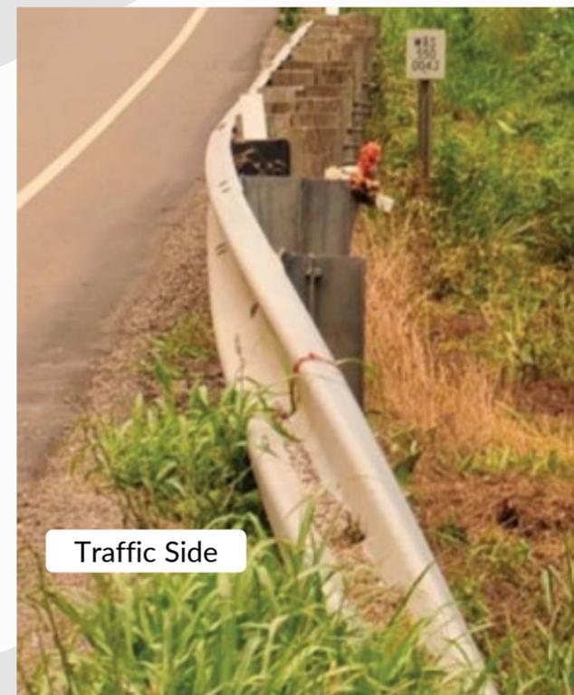
Differs from a buried terminal. Rail elements are not turned down for buried terminals and are attached to anchors buried in embankment.
