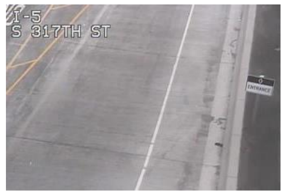
HOV Entrance sign located on the right side at the beginning of each on-ramp.
