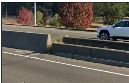
Photo A: Need for Mitigation - Single Slope Barrier Adjacent to Shorter Bridge Barrier
