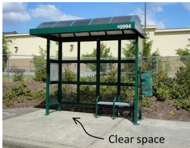
Passenger shelter showing clear space
