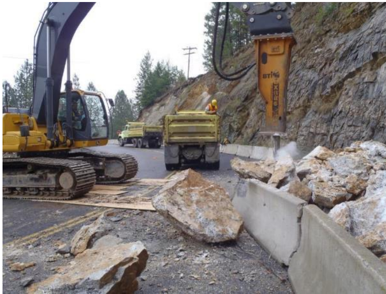
Maintenance clearing highway from rockfall overburdening catchment area
