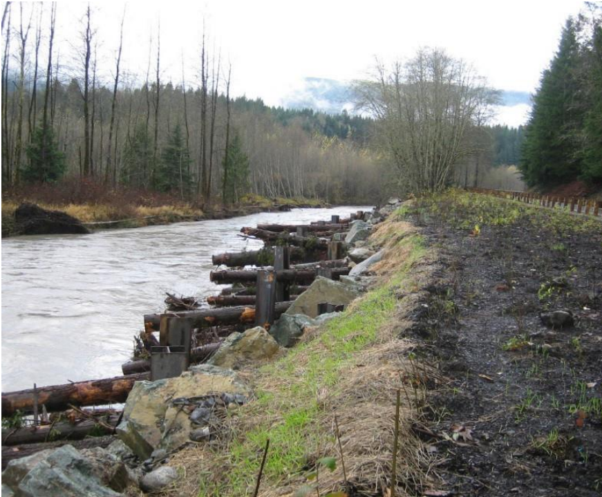
Figure 10A-5 Crib Wall with Steel Piles, Sauk River Side Channel, Skagit County
