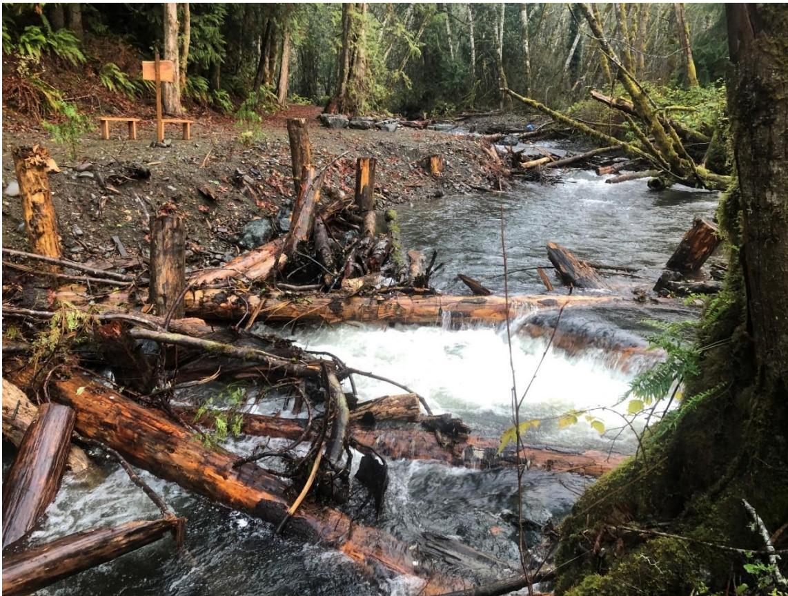
Figure 10-6 Example of Small-Channel Complex Log Grade Control
