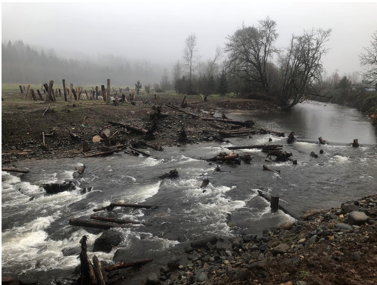
Figure 10-8 Example of Large-Channel Wood Grade Control
