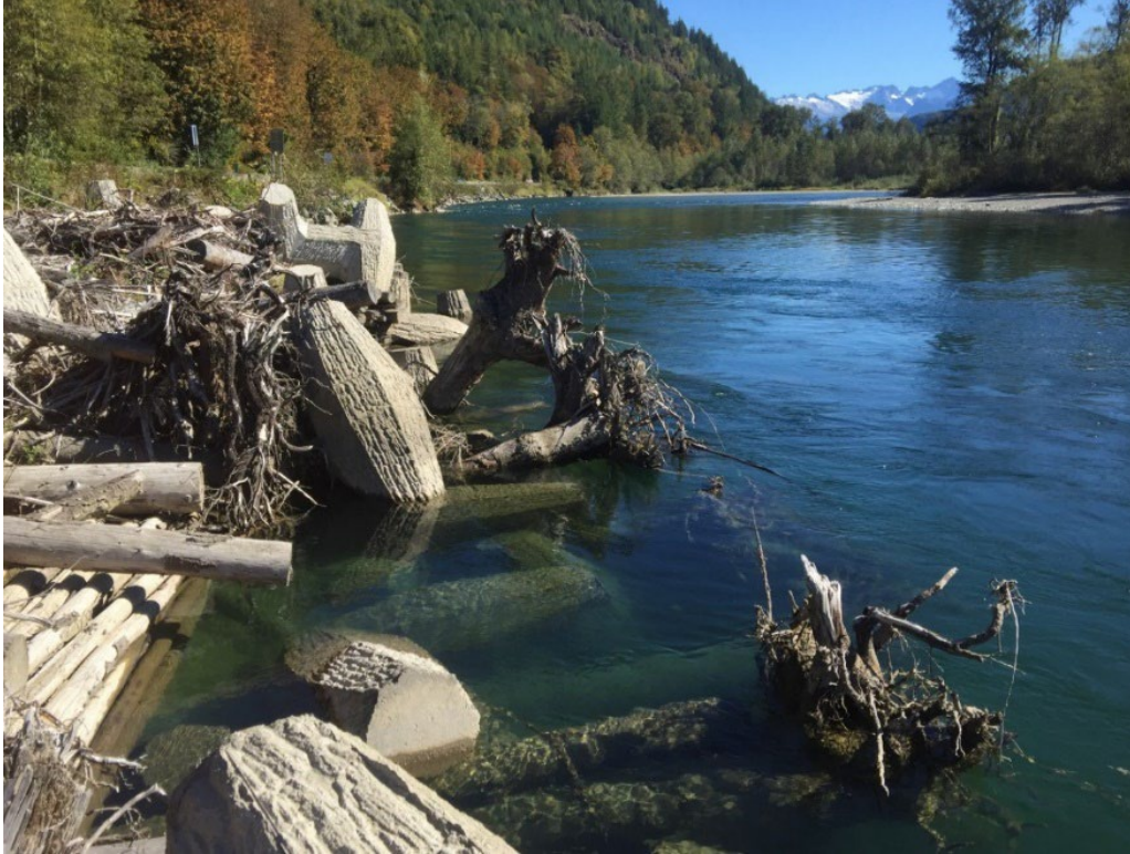
Figure 10A-9 Dolotimber Structures, Skagit River, Skagit County
