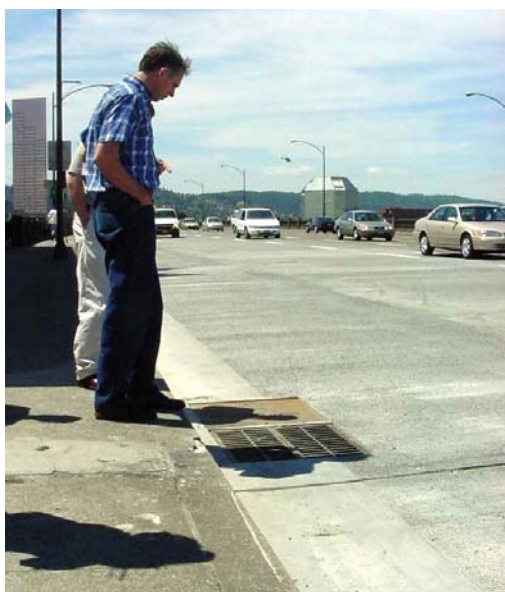
Figure RT.18.3. StormFilter™ catch basin in a bridge deck. (Courtesy Stormwater Management, Inc.)
