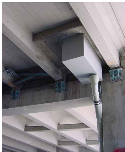
Figure RT.18.4. StormFilter™ catch basin in a bridge deck from under the bridge. (Courtesy Stormwater Management, Inc.)
