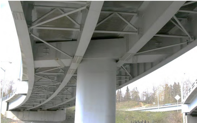
Figure 71. Curved bridge with curved girders. (Source: Alaska DOT)
