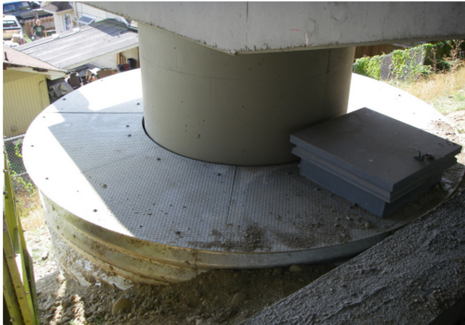
I-5 N-N RAMP OVER I-5 - 5/628N-N - 0016991A
