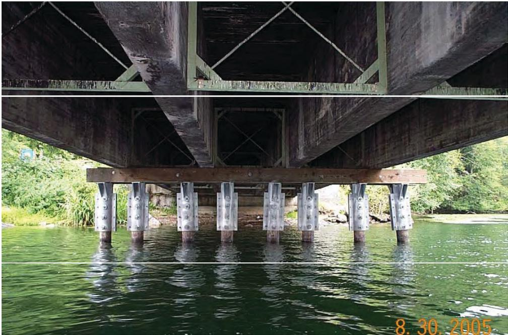
Photograph 4 : Steel brackets with newer crossbeam at Bent 5 looking south.
