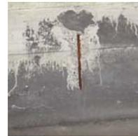
4. Length of truss affected with damage in significant locations or quantity and has reduced the structural capacity of the element or the bridge. Structural analysis is warranted or has determined repairs are essential to restore the full capacity of the element.
