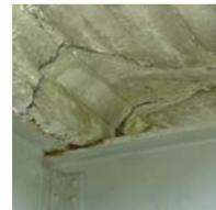
3. Deck soffit area showing signs of reduced structural capacity. Typical indications include areas with heavy to severe rust staining from deck reinforcement; Spalling with corroded rebar indicating active corrosion; Cracks that are full depth, severe, or leaking water.
