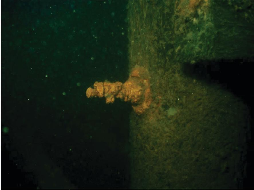
Photograph 5 : Typical condition of bolted connections prior to Level II inspection.
