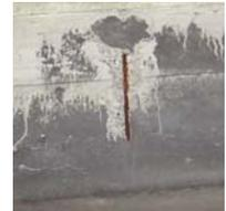
4. Girder span length with damage in significant locations or quantity and has reduced the structural capacity of the element or the bridge. Structural analysis is warranted or has determined repairs are essential to restore the full capacity of the element.
