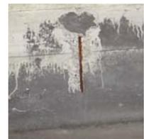
4. Floorbeam span length with damage in significant locations or quantity and has reduced the structural capacity of the element or the bridge. Structural analysis is warranted or has determined repairs are essential to restore the full capacity of the element.
