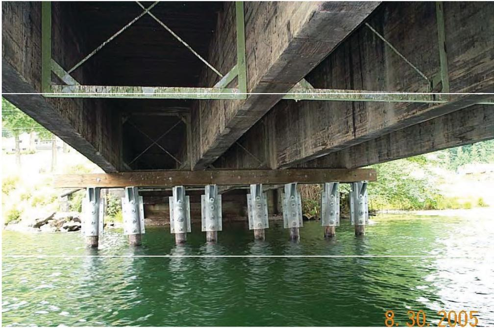
Photograph 1 : Steel brackets with newer crossbeam at Bent 2 looking south.
