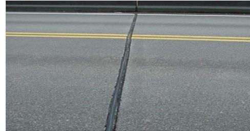
**405      Compression Seal/Polymer Header****Units - LF**
