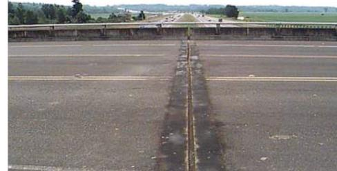
**406      Compression Seal/Steel Header****Units - LF**
