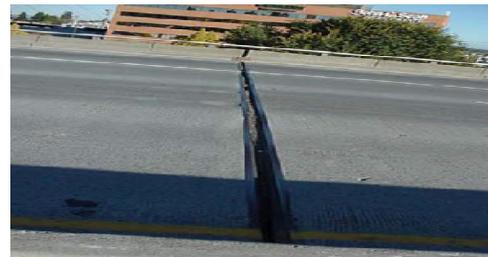
**414 Bolt Down - Sliding Plate w/springs****Units - LF**
