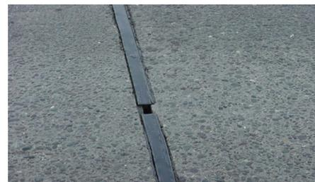
**404      Compression Seal/Concrete Header****Units - LF**
