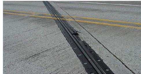
**416 Assembly Joint Seal (Modular)****Units – LF**
