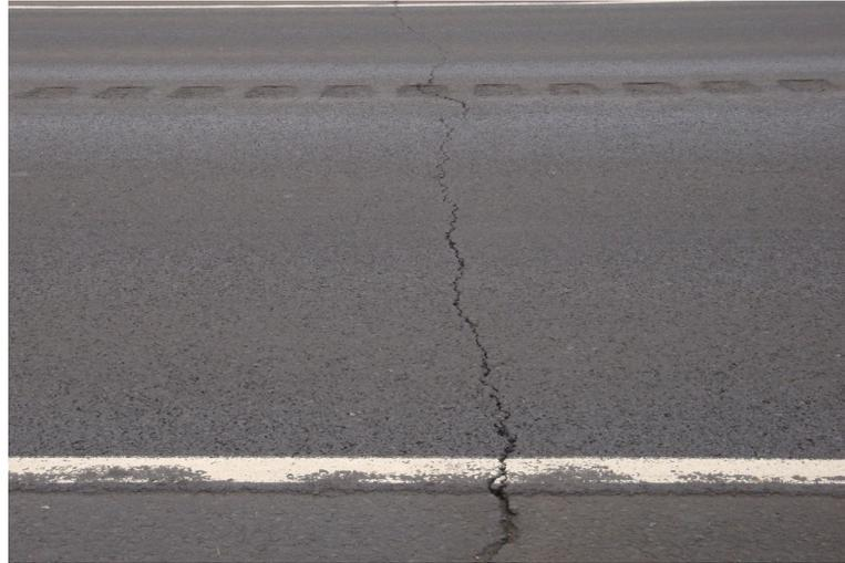
Transverse cracks are most typically a working crack and sealing these cracks with a rubberized material is the most effective treatment option, although crack sealing is an alternative if a mastic material is used.
