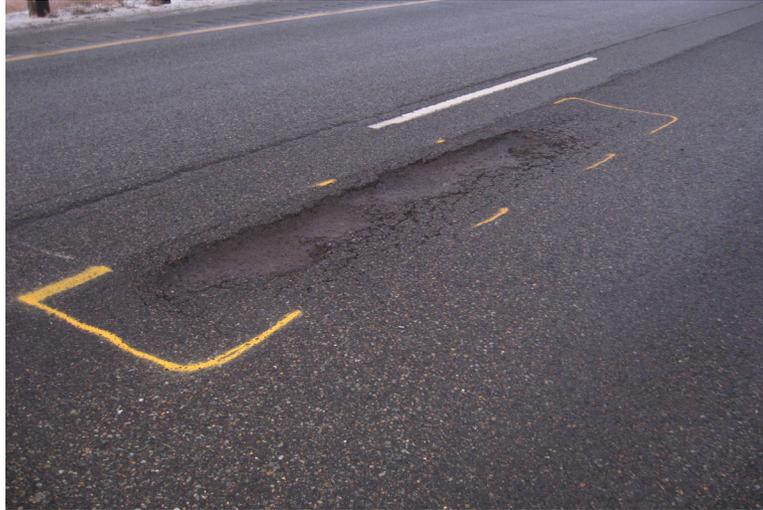
Pothole repairs will generally be full-depth patches but care should be taken to confirm that they are full-depth. The repair area will always need to extend beyond the limit of the visible distress in order to get to sound material. If repairs only include the affected area, reoccurring distresses typically result.
