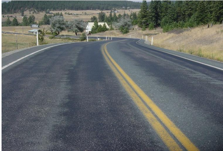
Removal and replacement of flushed or bleeding pavement areas is an expensive, but sometimes cost-effective method of repair. Another option is to perform a chip seal with minimal or no emulsion but this approach necessitates proper prior planning. If repairs are not possible prior to a seasonally wet period, contact the regional traffic engineer to evaluate friction and the need for posting “Slippery When Wet” signs.
