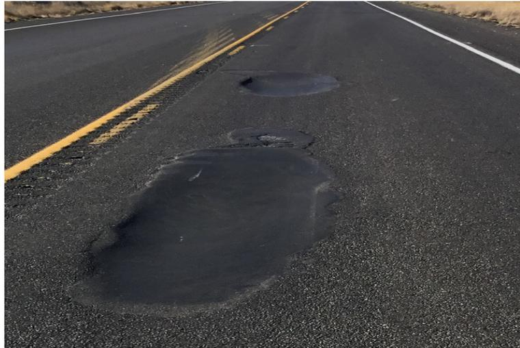
This distress typically results in full-depth repairs although a partial-depth patch or a micro-grind may be used depending on the cause of the distress.
