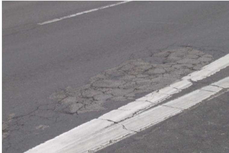
If the alligator cracking isn't extensive, subgrade material isn't visible and signs of depressed pavement isn't present, a chip seal might be a possibility. The typical repair method, however; is to complete a partial-depth or full-depth patch. Full-depth cracking extends through the entire pavement structure, whereas partial-depth cracking goes through a portion of the pavement.
