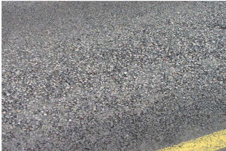
The best treatment option for a pavement that is raveling or pitting is to perform a fog seal to ensure the pavement has been sealed and thereby reduce the rapid deterioration usually exhibited from this distress. If raveling becomes severe a chip seal is an alternative.
