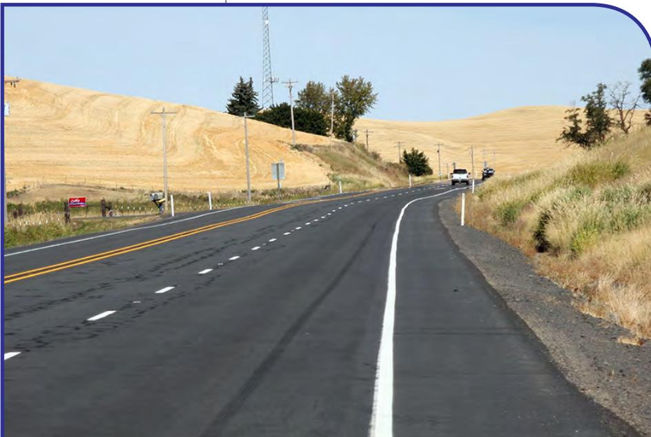
*Passing lanes are often constructed on two-lane roadways to improve overall traffic operations by breaking up traffic platoons and reduce delays caused by inadequate passing opportunities over substantial lengths of roadway.*
