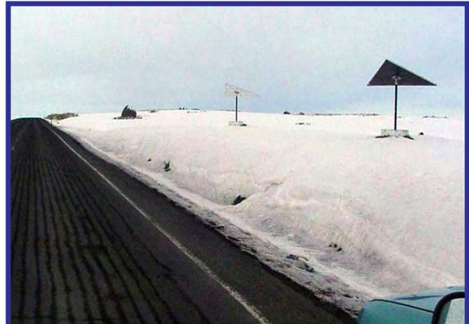
*Pivoting in the wind, vortex generators redirect the natural airflow to clear the highway of snow on State Route 172, near Mansfield.*
