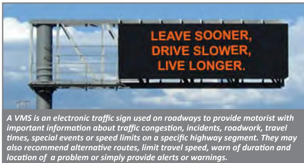
A VMS is an electronic traffic sign used on roadways to provide motorist with important information about traffic congestion, incidents, roadwork, travel times, special events or speed limits on a specific highway segment. They may also recommend alternative routes, limit travel speed, warn of duration and location of a problem or simply provide alerts or warnings.
