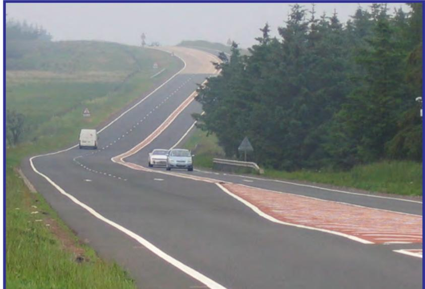
*This 2+1 passing design configuration has a continuous three-lane cross section with alternating passing lanes.*
