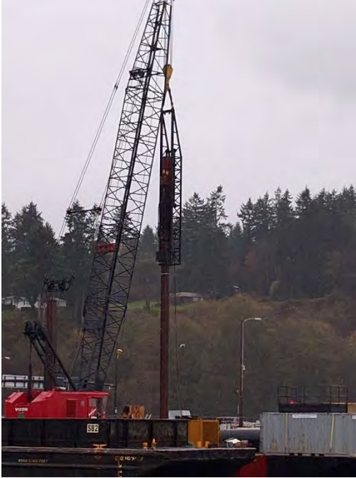
Figure 3a. The placement of the impact hammer on the control pile, taken from the R/V Robertson on 7 December.
