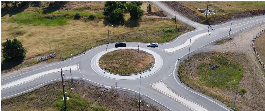
Glenrose Rd & Carnahan Rd Safety Improvements (2019) Spokane County
