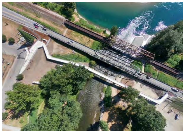
Sultan River/US 2 Bike and Pedestrian Bridge (2022)
