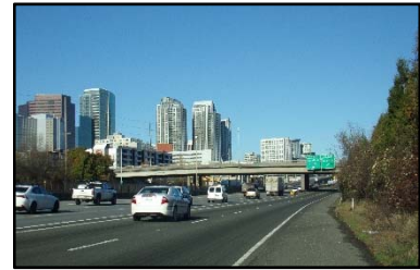
Existing Main Street Overpass
