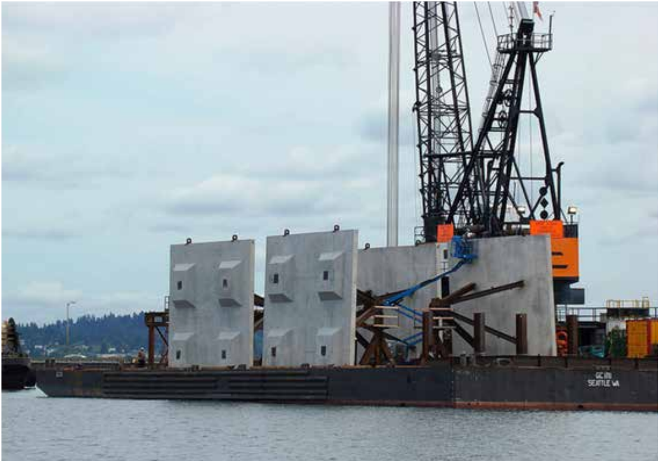
Completed fluke anchors are barged from Kenmore to the bridge-assembly site on Lake Washington. The graphic below shows how fluke anchors are placed in the lakebed.
