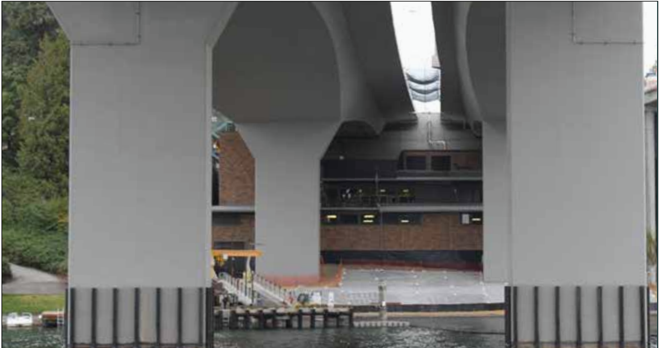
Bridge maintenance facility and dock: A LEED-certified bridge maintenance facility and dock under the east approach of the bridge give maintenance staff improved access to the floating bridge.
