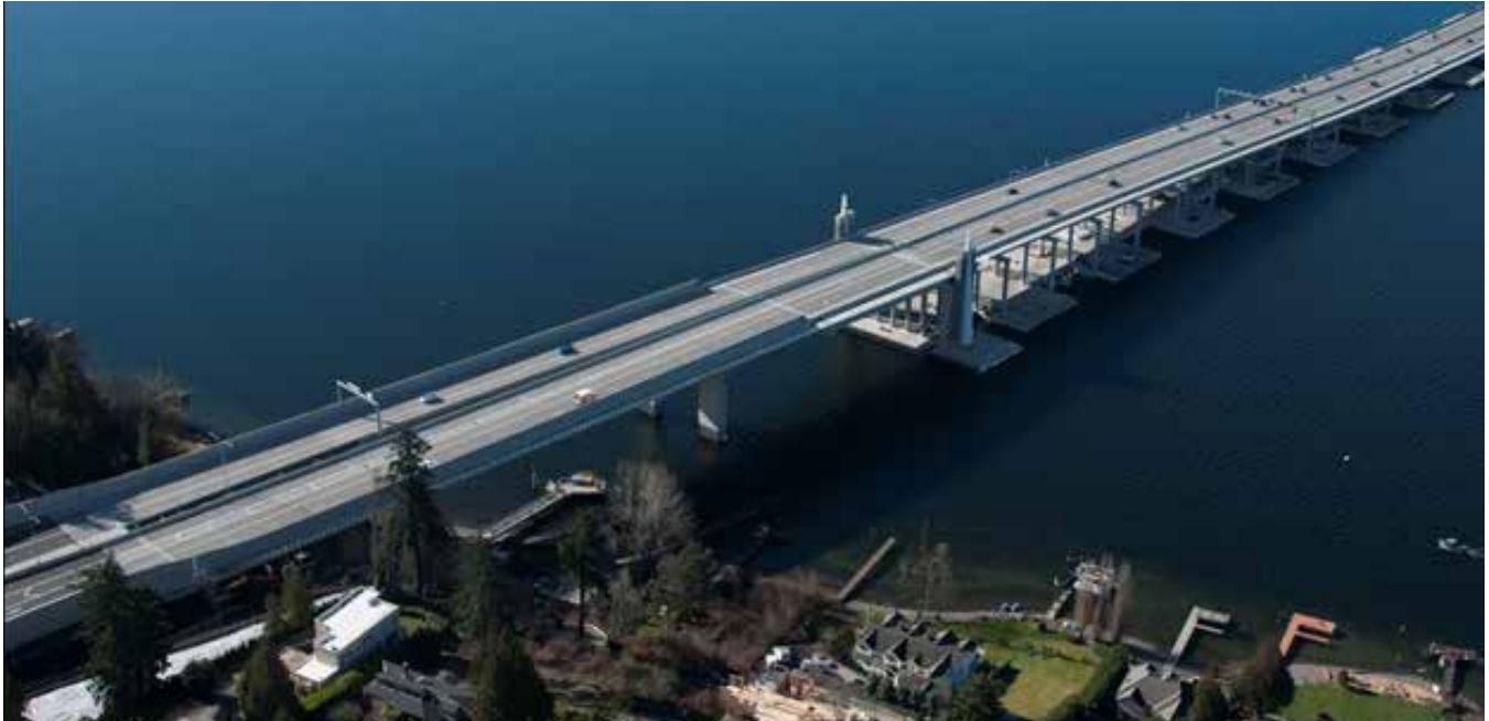
Approach bridges: This photo shows the two east approach bridges (at left) – one for westbound traffic, one for eastbound traffic – that connect to the new floating bridge near Medina. WSDOT also is building two new west approach bridges between the floating bridge and Seattle.
