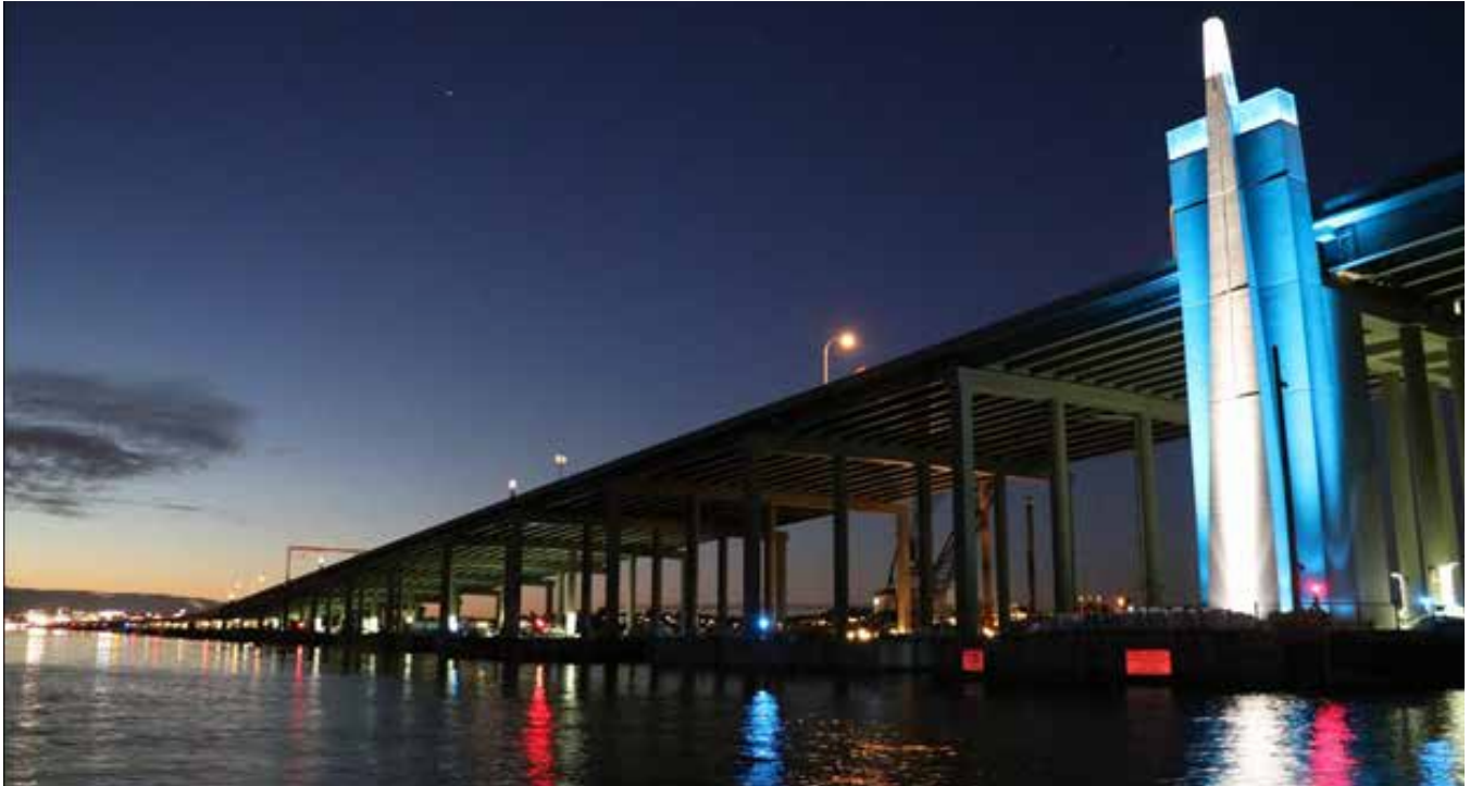
Sentinels: Four sentinels mark the transition between the floating bridge and its fixed approaches at the east and west ends. The LED lights in the sentinels feature numerous color options.
