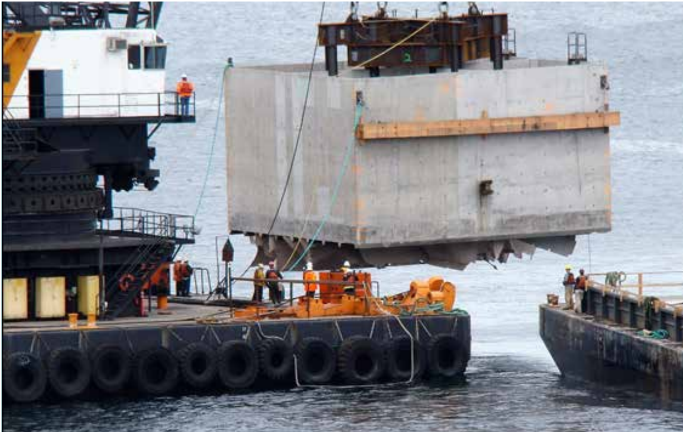
Workers aboard a derrick barge lower a 420-ton gravity anchor into Lake Washington.
