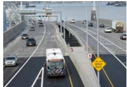
A view of the new floating bridge just after it opened to traffic in April 2016.
