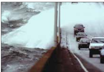
Waves batter the old SR 520 floating bridge – and traffic – during a storm.
