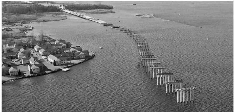
Construction of the old SR 520 floating bridge west approach on Lake Washington on March 20, 1962. Courtesy Seattle Municipal Archives (Image No. 70342). View more historical images at 520history.org
