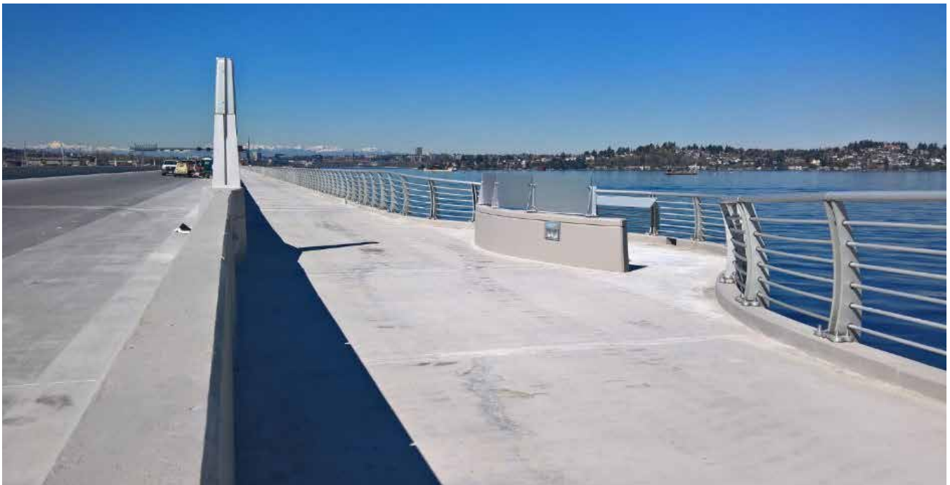
Railing: The bicycle and pedestrian path has 8,425 feet of specially designed railing to both keep people safe and allow unrestricted views of north Lake Washington.
