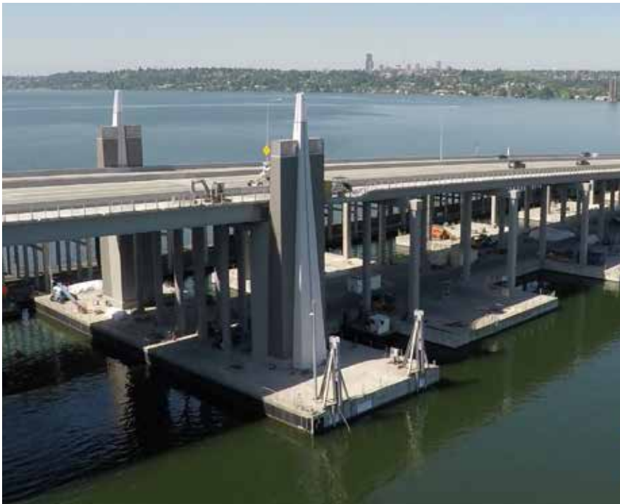
The new bridge has more than twice as many support pontoons.
