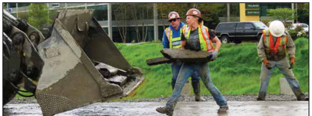
SR 520 construction workers do some heavy lifting during a highway closure.
