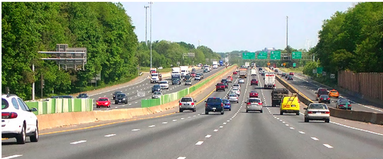
I-495 Capital Beltway in Virginia.
