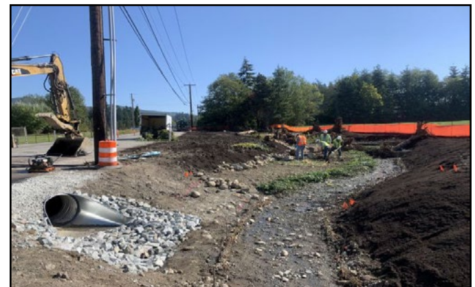
Figure 14. Top (CR2): Concrete box culvert, 12.3 ft span, and 13.5 ft rise.
