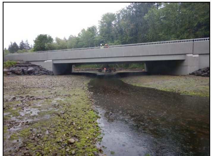
Figure 36. The new crossing is a 70.5 ft concrete girder bridge, improving access to 0.82 miles of potential habitat for chum, Chinook, coho, steelhead, coastal and resident cutthroat trout to the SR 16 crossing.
