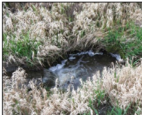
Bottom (995265): Round corrugated steel culvert 2.5 ft in diameter and 222.1 ft long.
