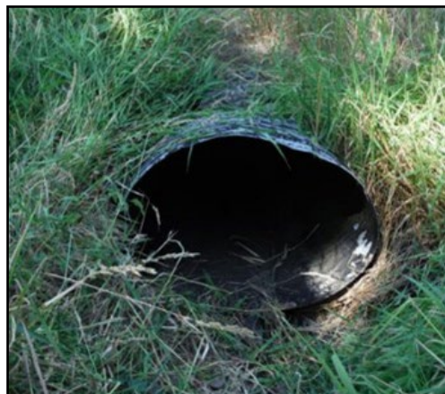
Figure 25. Top (991225): Old crossing was a 4.6 ft span by 3.3 ft rise squash, corrugated steel culvert. This site was a barrier due to an excessive hydraulic drop.
