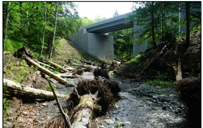
Figure 8. The new crossing is a 73.8 ft span concrete girder bridge.
