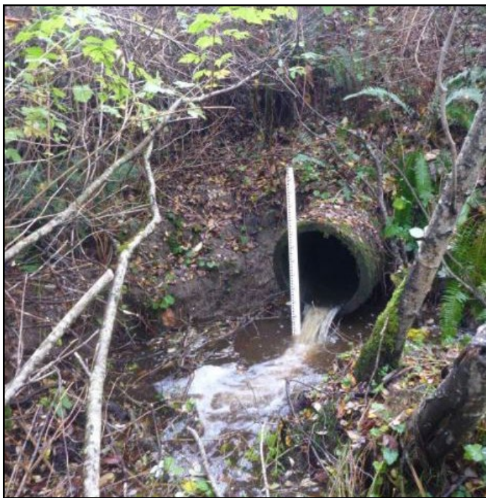
Figure 42. The old crossing was a 97 ft long, 2 ft diameter concrete culvert.
