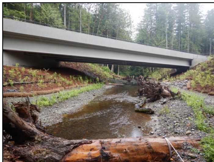
Figure 52. The new crossing is a 117 ft concrete girder bridge. An adult coho salmon was video recorded swimming under the new bridge in September 2023.
