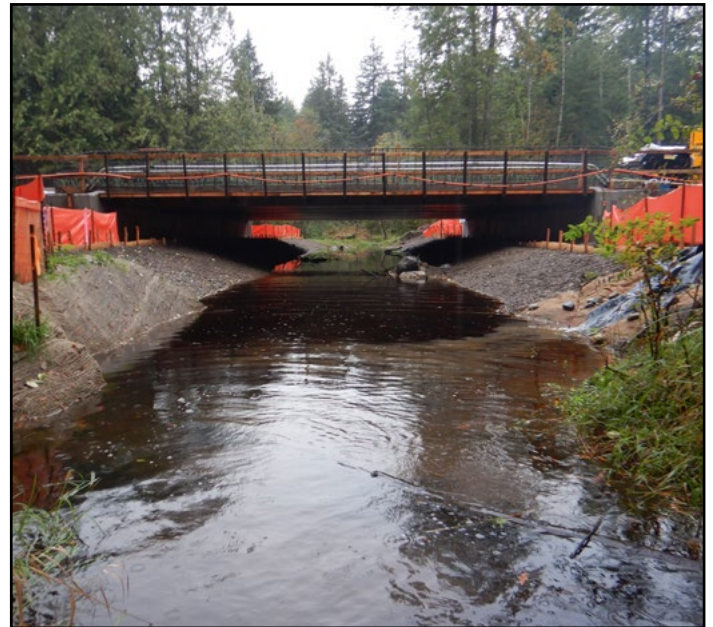
Figure 18. The new crossing is a 43.7 ft span concrete bridge.
