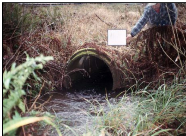
Figure 57. Top (993702): The old crossing was a 3 ft diameter concrete culvert that was a barrier due to slope. Bottom (993704): The old crossing at 993704 was also a 3 ft diameter concrete culvert that was a barrier due to slope.
