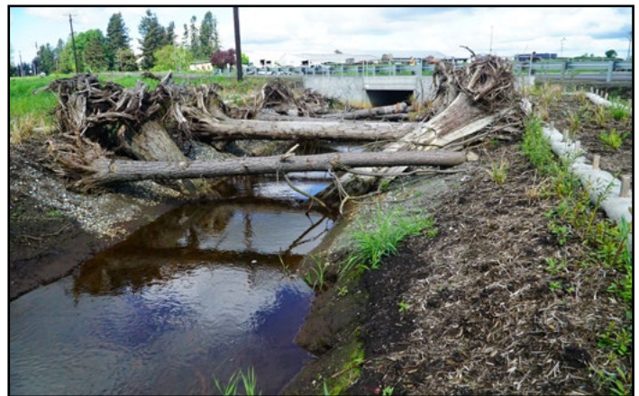
Figure 10. The new crossing is a concrete box culvert with a span of 12.2 ft and a rise of 10 ft.
