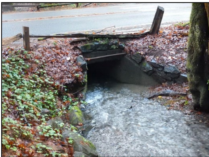
Figure 27. The old crossing was a 4 ft span by 4 ft rise concrete box culvert that was a barrier due to velocity.
