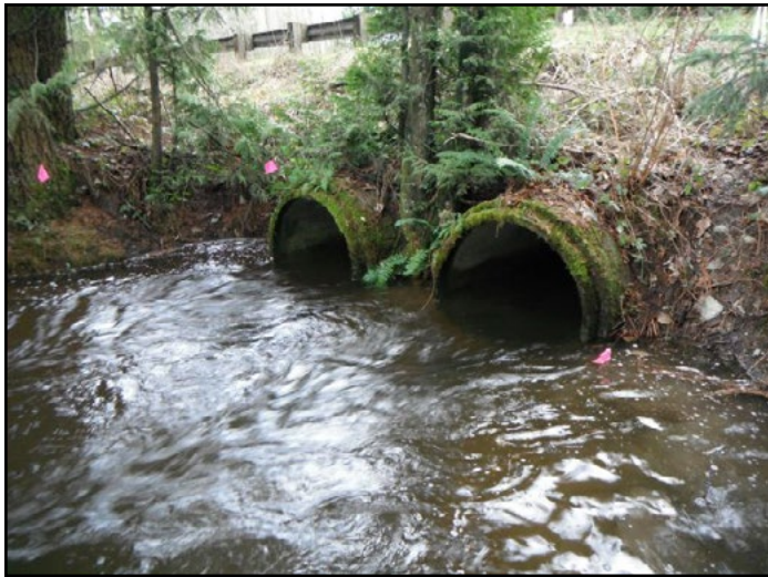
Figure 17. The old crossing was a 3.5 ft diameter round concrete culvert.
