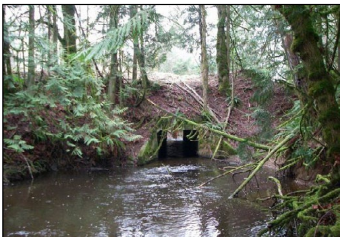
Figure 50. The old crossing was a single cell concrete box culvert measuring 8 ft span, 6 ft rise, and 145 ft long. The culvert was a barrier due to excessive water velocity.
