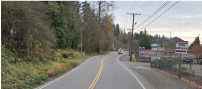
East Valley Highway
