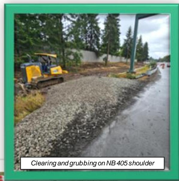
*Clearing and grubbing on NB 405 shoulder*
