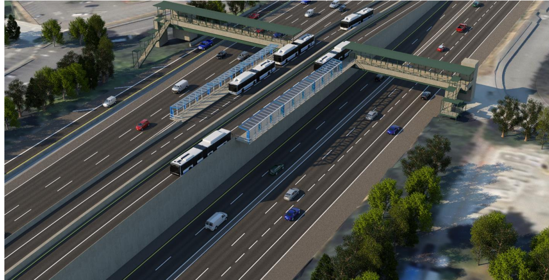
Aerial view of the future Stride in-line station on I-405.
