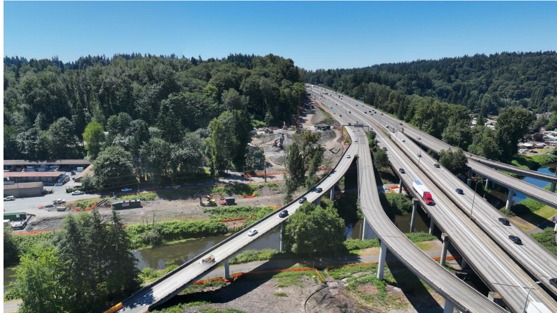
Looking south, location at NB I-405 on-ramp to SR 522
