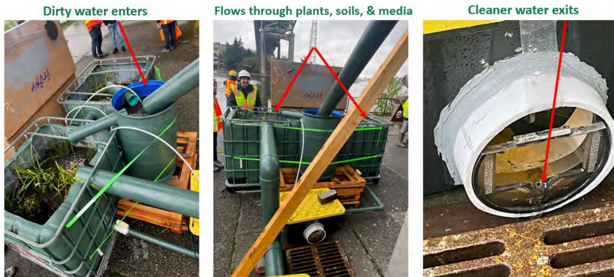
Adopt-a-downspout stormwater treatment test project.
