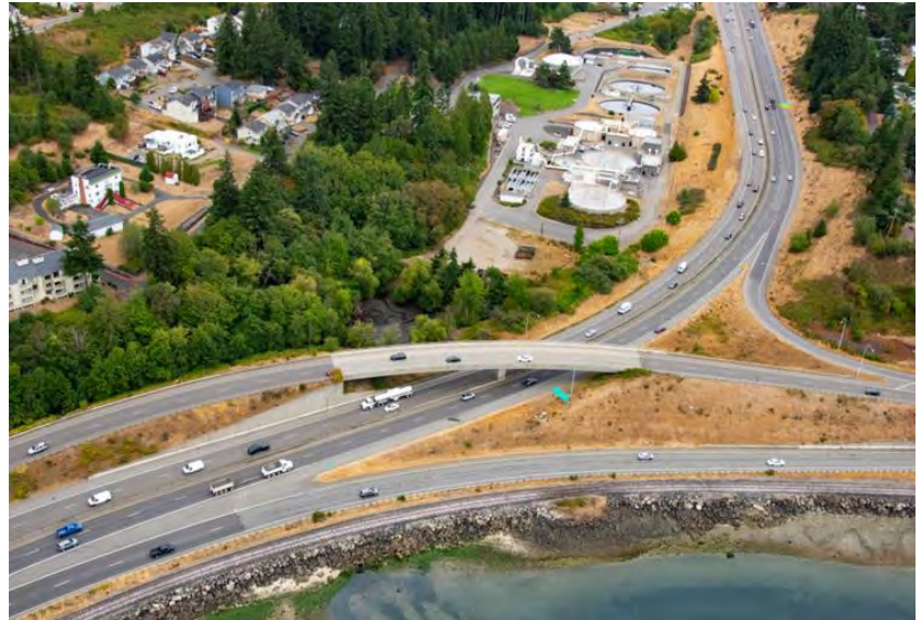
Charleston Boulevard overpass at SR 3.
