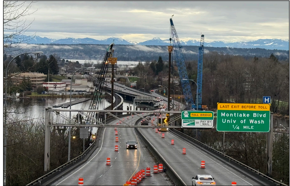
Recent weekend single-lane closures on SR 520.
