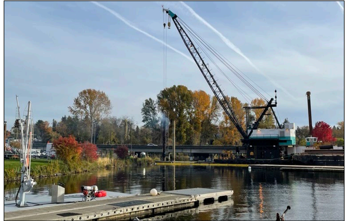
Crews using an impact hammer to install piles in Portage Bay.
