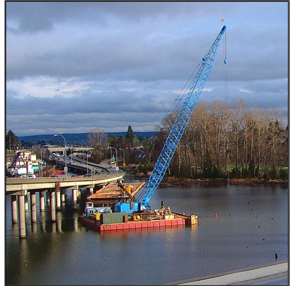
Image of the current in-water work barge.
