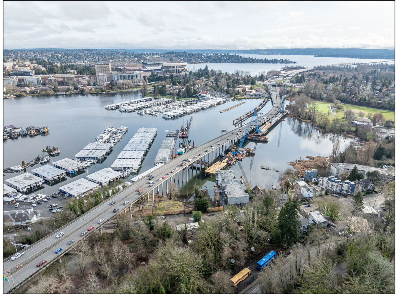
Aerial image of Portage Bay Bridge construction.
