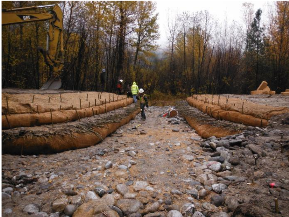
Photograph 12 Completed installation of FESL looking downstream
