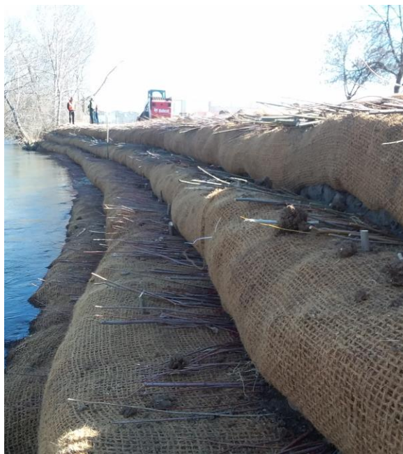
Photographs 1 and 2 Recently constructed FESL along the Boise River (looking upstream). Photos taken March 2019 (left) and August 2020 (right).
