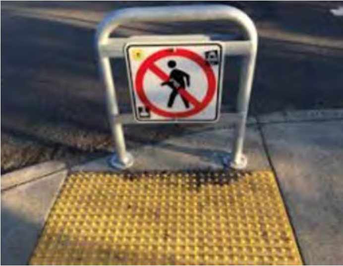
Physical Fence Barrier— max 15" above ground level
