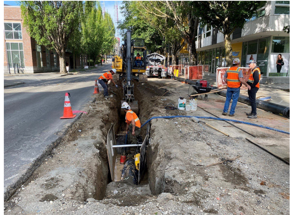
Crews dig a trench to place electrical lines underground. Photo credit: SDOT
