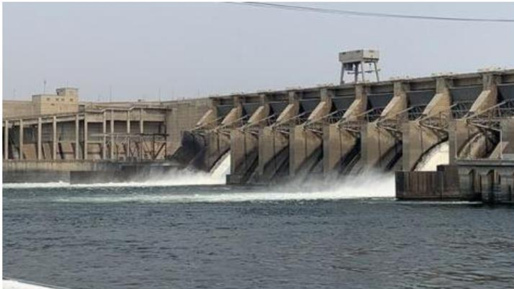
The Ice Harbor Dam on the Snake River in Washington. Courtesy: U.S. Department of Energy, Flickr
