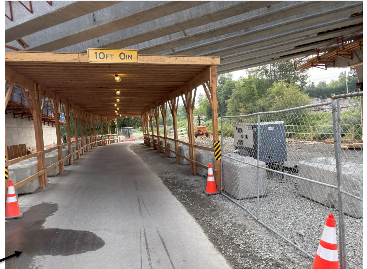
Pedestrian protection underneath the new I-405 northbound ramp to eastbound SR 522
