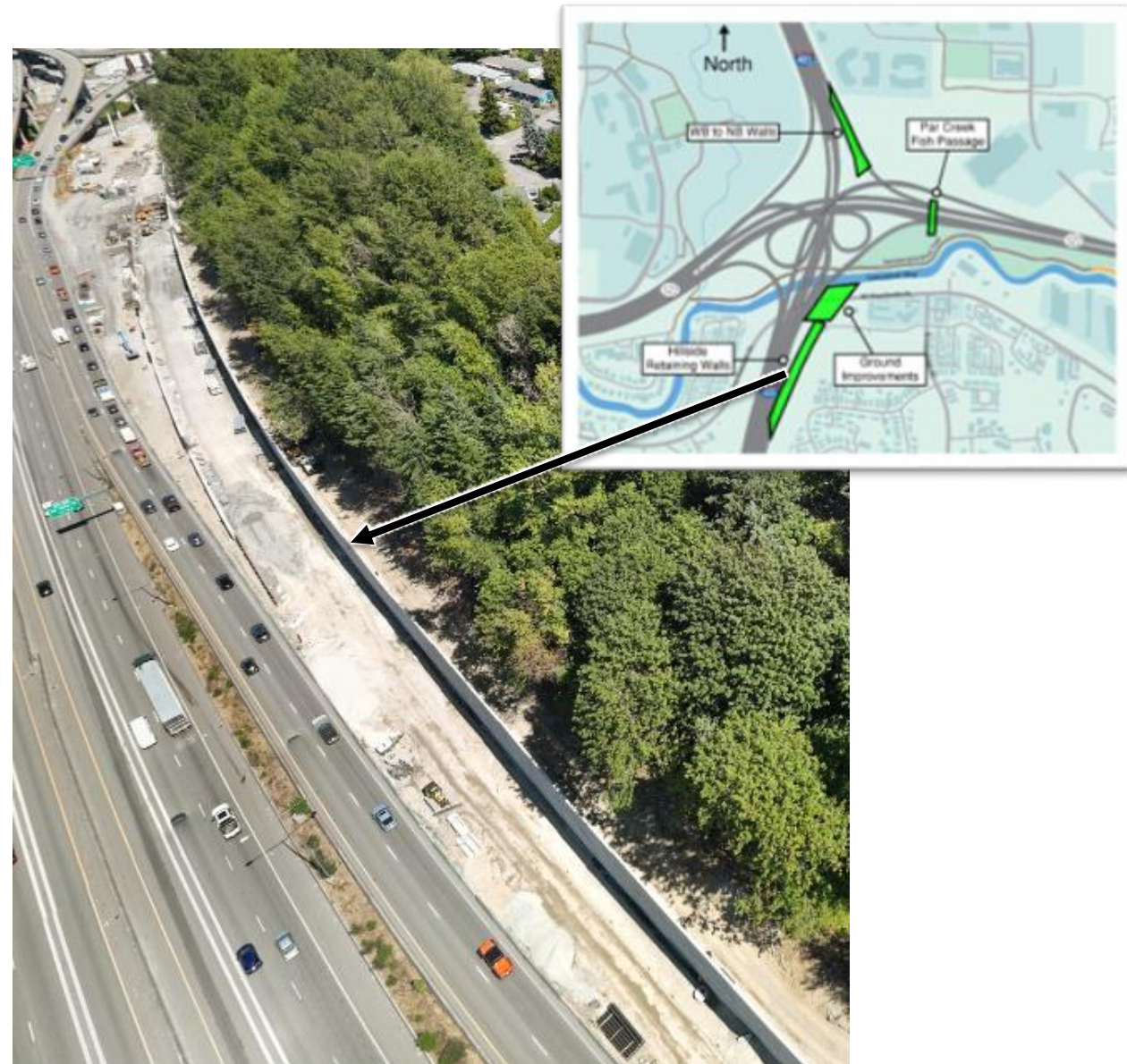
Looking northeast at tieback wall construction along northbound I-405
