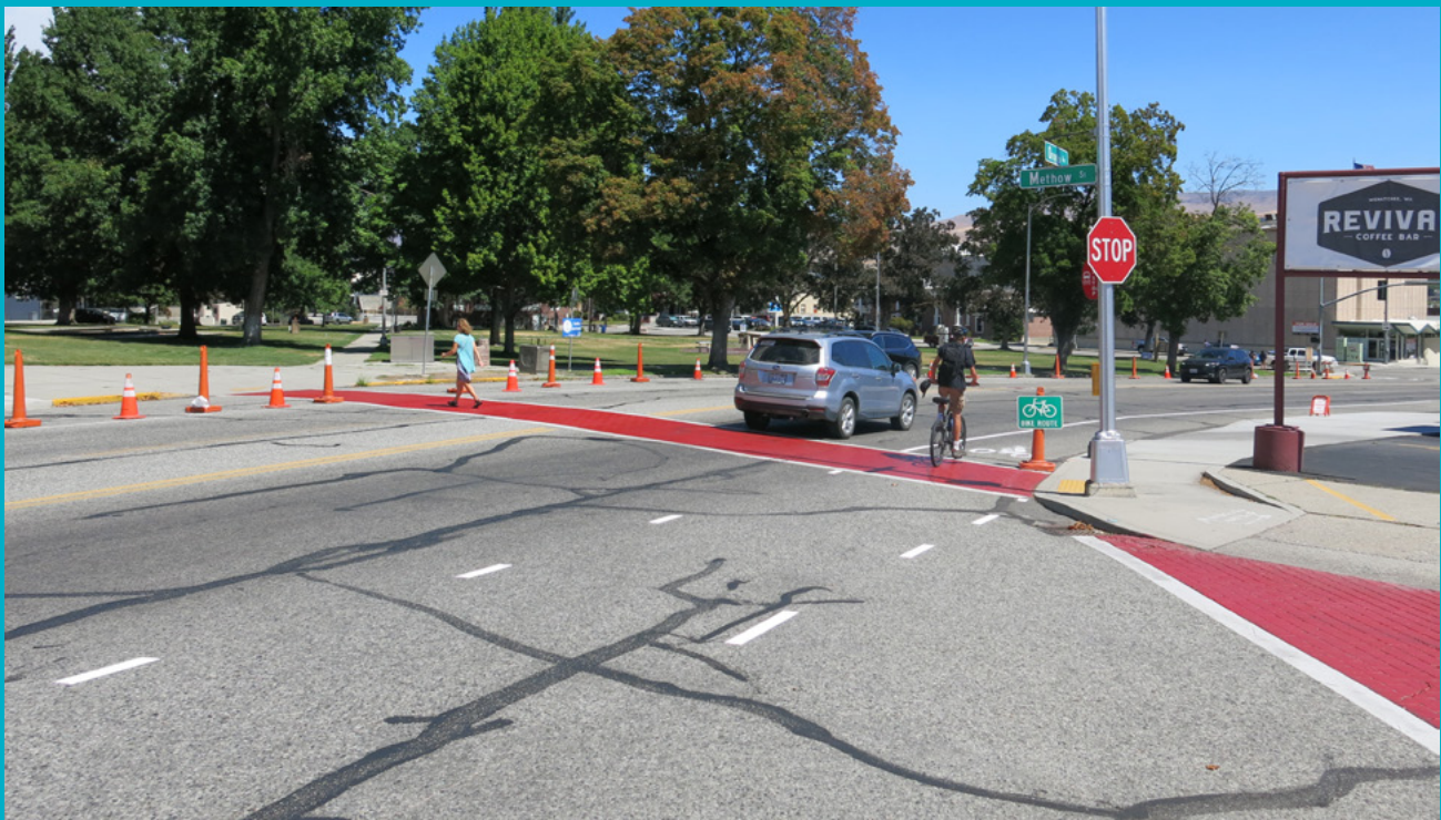
FIGURE 11 Intersection from a Demonstration project in Wenatchee, WA
