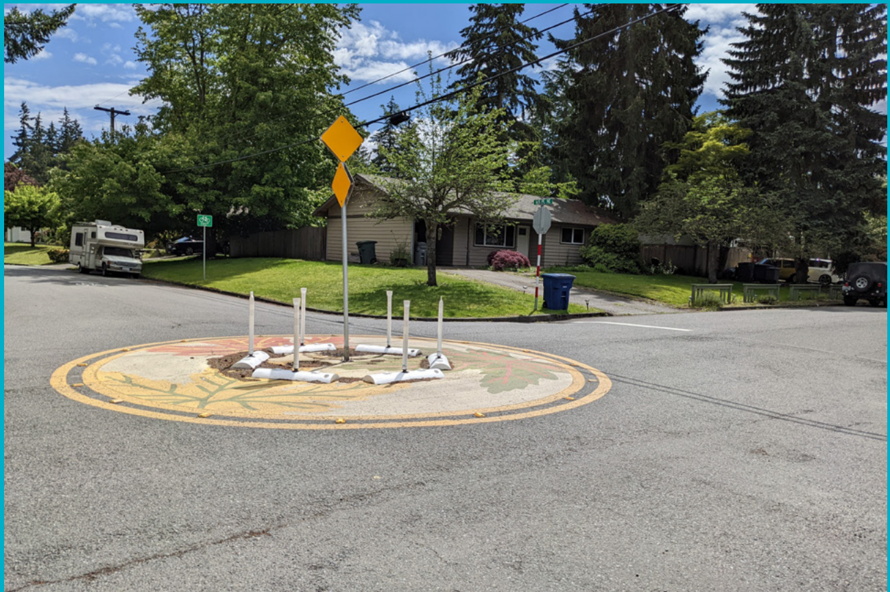
FIGURE 12 Thermoplastic marking used with delineators for a Pilot project at a traffic circle in Bellevue, WA
