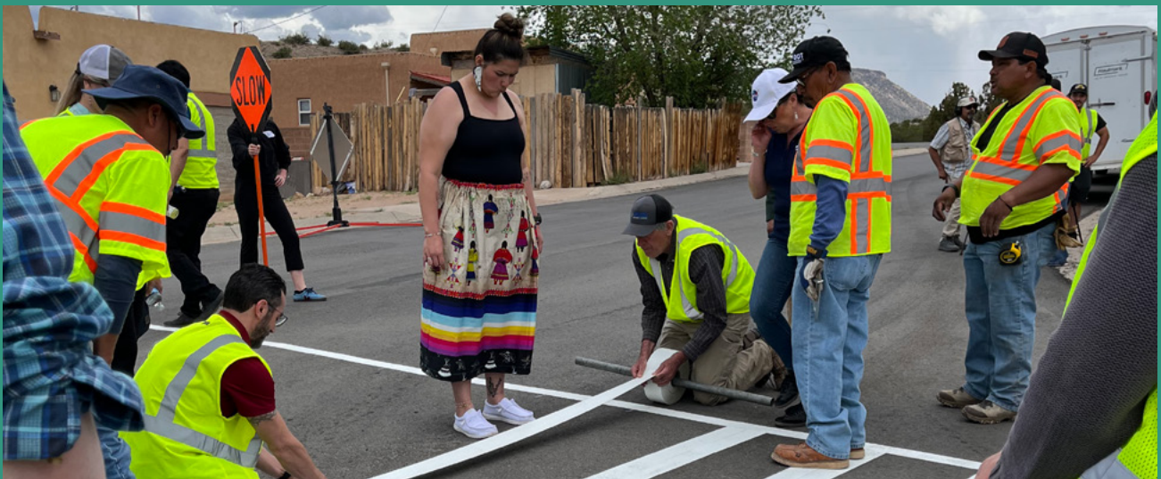
FIGURE 18 Installation of a Quick Build project in Pueblo of Jemez, NM
