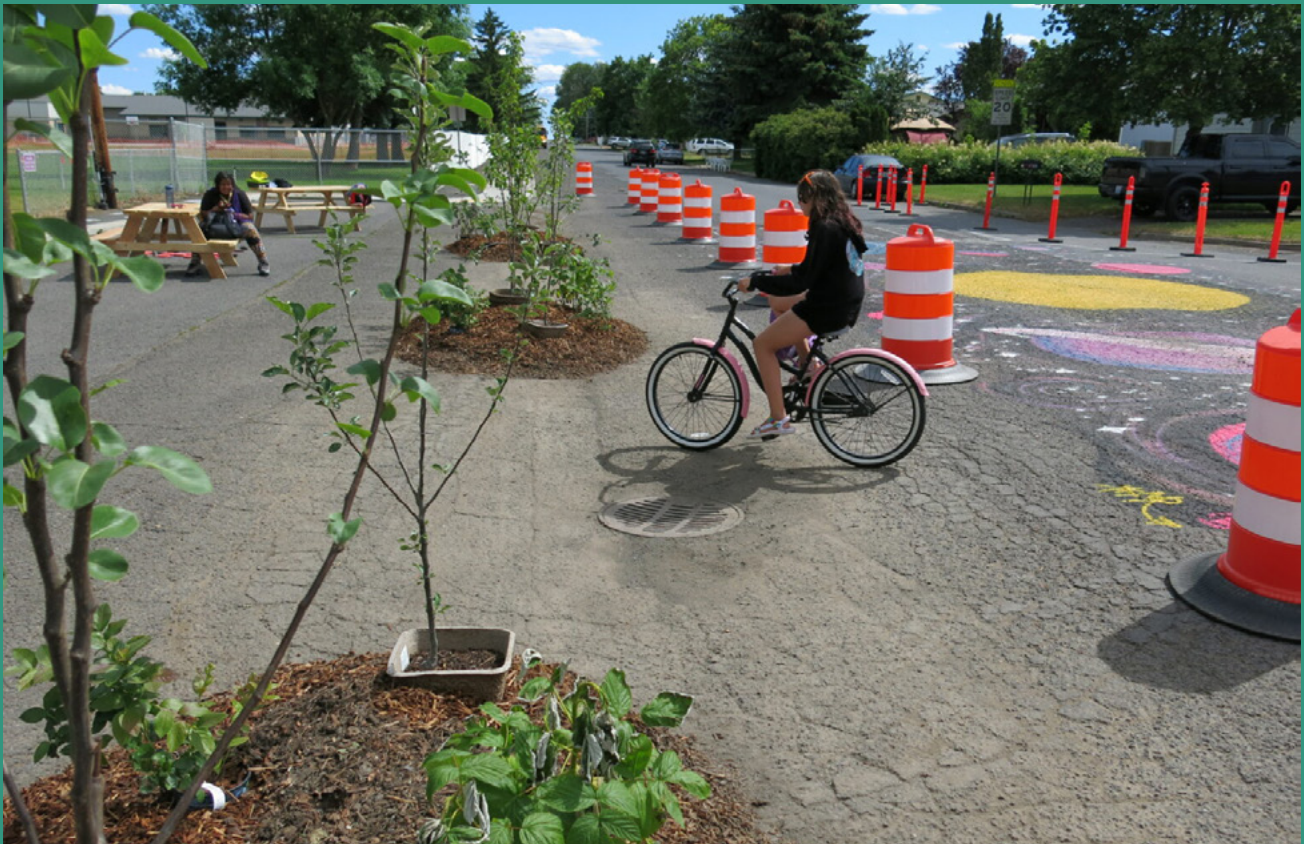
FIGURE 6 Traffic safety drums create a protected walkway for a safety Demonstration project in Airway Heights, WA
