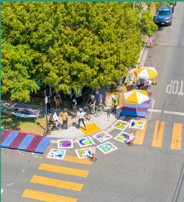
FIGURE 14 Demonstration curb extension in Long Beach, CA
