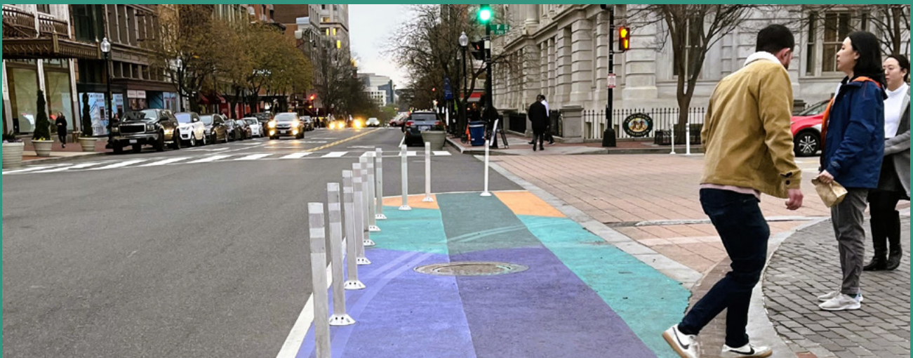
FIGURE 13 Curb extension from a Quick Build project in Washington, DC
